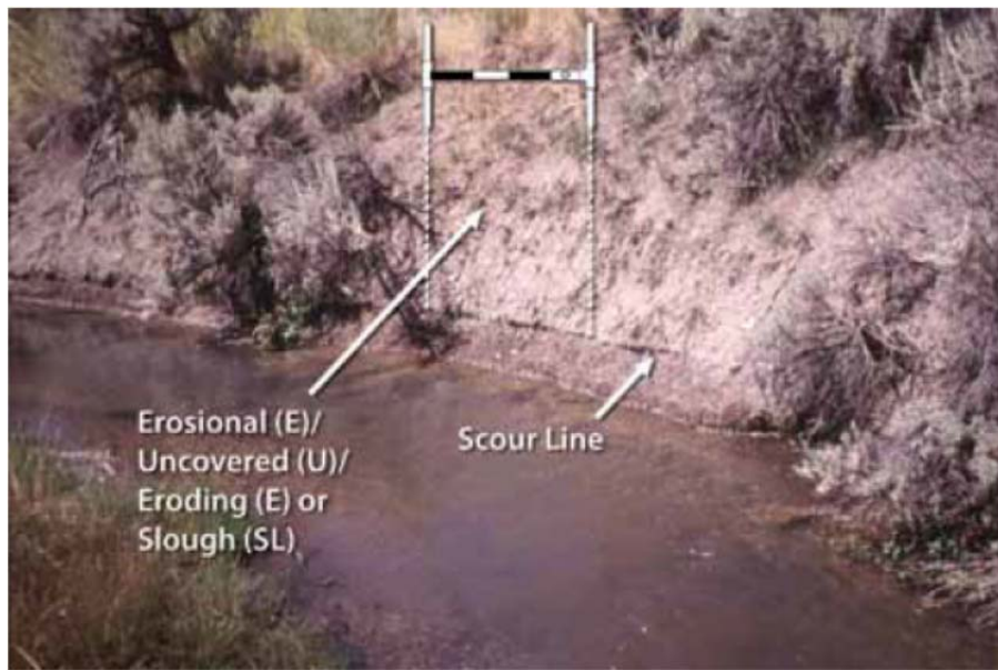
Fig. 21. The streambank has an obvious scour line. The bank evaluated is above the scour line to the first bench and is recorded as erosional (E), uncovered (U), and eroding (E) or slough (SL) (Burton et al. 2010).
